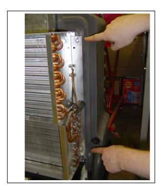
– Pull the back case back from top of coil – it will only move back about 6" but this is enough to get to the defrost sensor wire – see below
